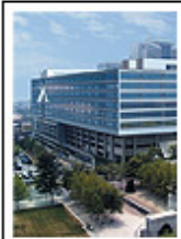
SunTrust Plaza Garden Offices Atlanta, GA
